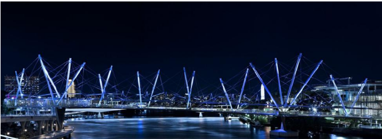
Figura 3. Puente Kurilpa, Brisbane, Australia (2009) [8].
