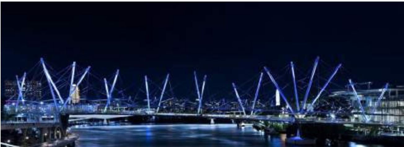
Figura 3. Puente Kurilpa, Brisbane, Australia (2009) [8].
